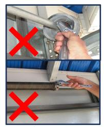
Forces generated in springs are generally equal to the door weight, and those forces are violently released if a spring breaks while wound.
